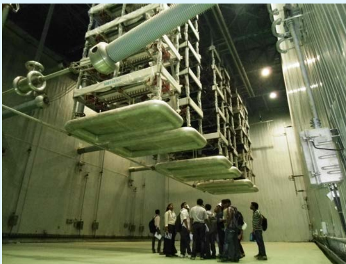
On Job Training at HVDC Station
