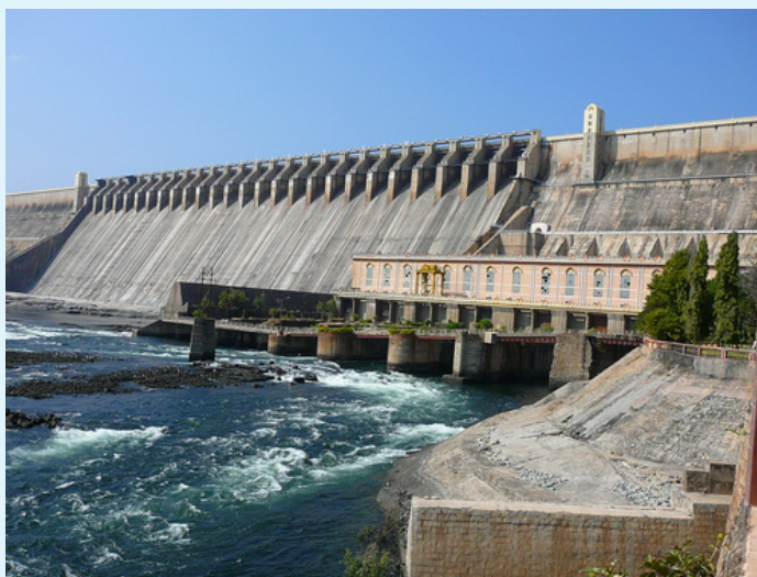
Hydro Power Station
